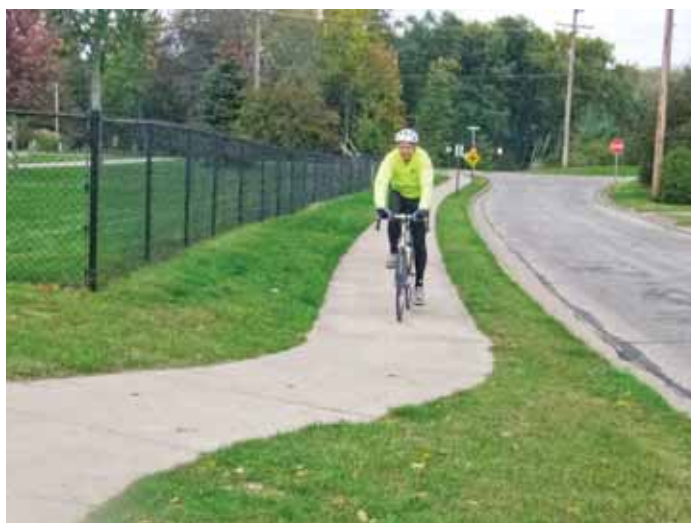
Before, looking north: The four-foot “sidewalk” along Railroad Street in Middlebury was too narrow for bikers to pass. (Photo by John Yoder)
